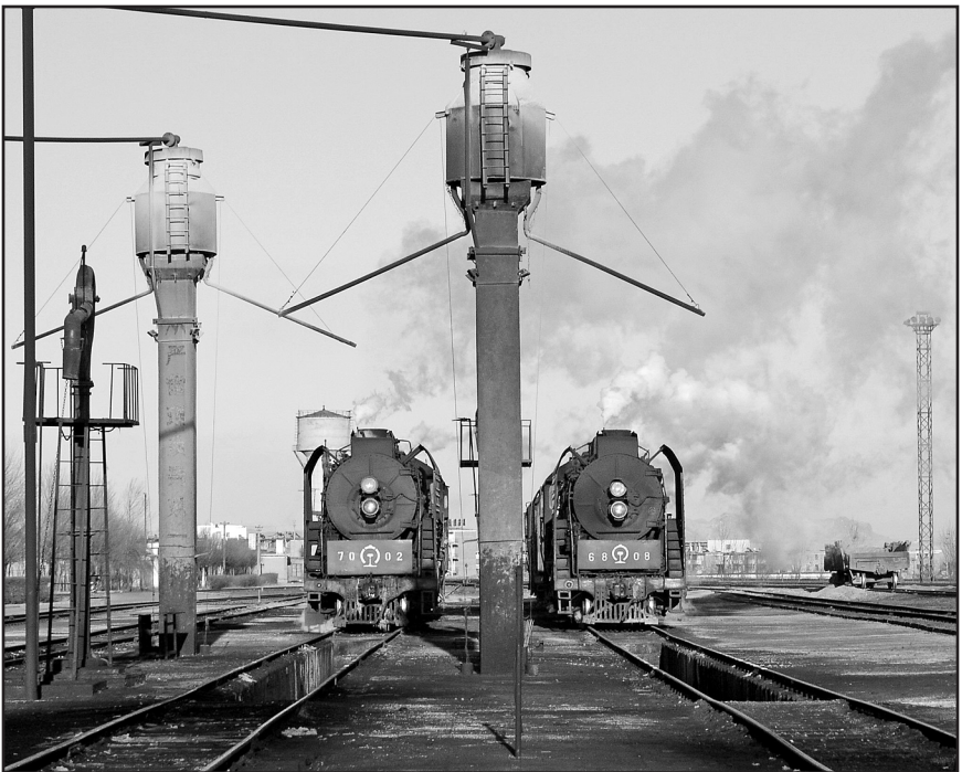
A small part of the Daban engine servicing facilities in March 2004. – Photo © 2004 Keith Jensen.
